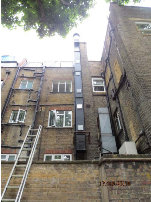
Pre-existing extract duct
